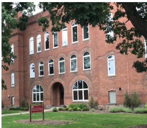
The newly renovated Academic Building, with the Constantakis namesake
